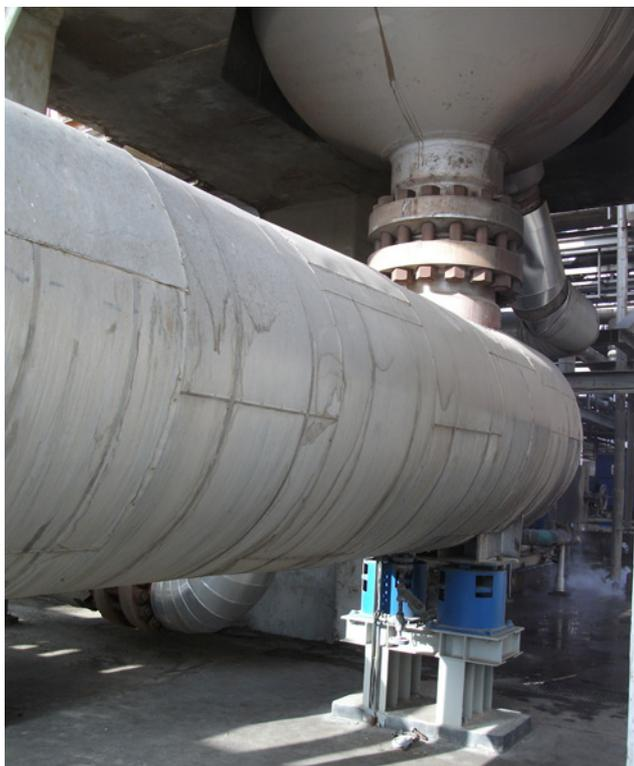
**Figure 6.** Direct connection between converter and hot heat recovery exchanger.
