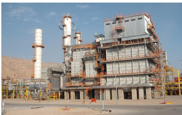
**Figure 3.** Primary reformer in a 2050 tpd ammonia plant.
