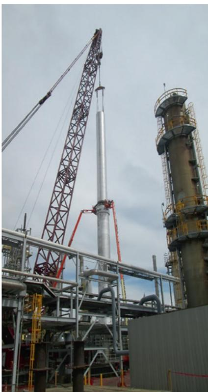
*Fig. 7: Cartridge lift and installation inside converter.*
