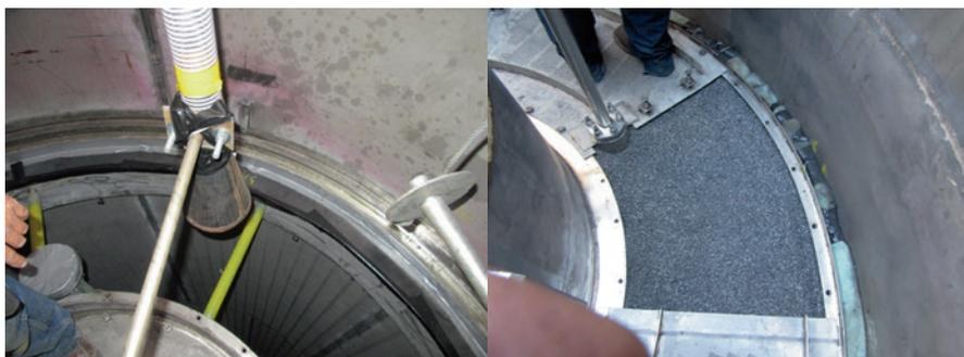
Fig. 9: Catalyst dense loading.
